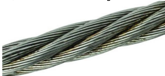
Heat, Chemical or Electrical damage
