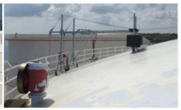
The ElectroGas Malta tank farm is the largest in Malta and provides the majority of gas supplies on the island. Sky Climber was selected by the maintenance contractor to develop a suspended access system to allow service and maintenance to be carried out on the vertical surfaces of the tanks. The suspended platform is used to clean, paint and repair the steel casing of the tanks.
