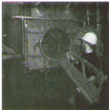
8:10am Pass components through tight 18" access into work area.
